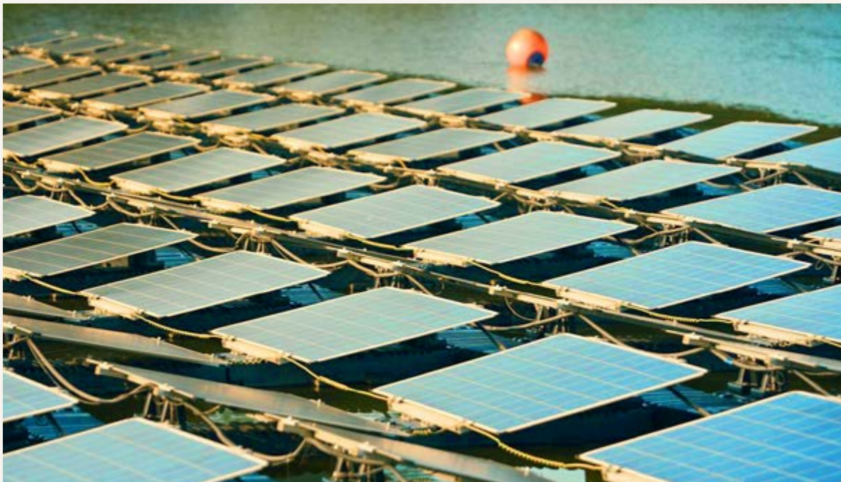
Singapore has one of the world's largest floating solar panel farms, about the size of seven football fields.
